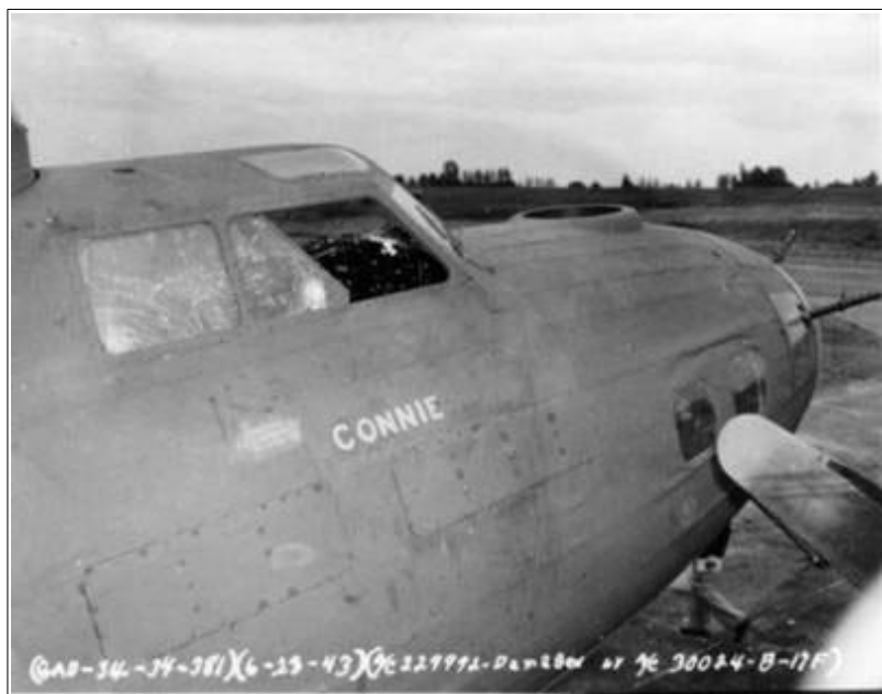
Lt. Carah's Original B-17F 42-29992 (OQ-J) 23 June 1943. Nearby Bomb Loading Accident Destroyed the Aircraft "Connie," Named after his Wife. Note Blown Off Astro Dome
